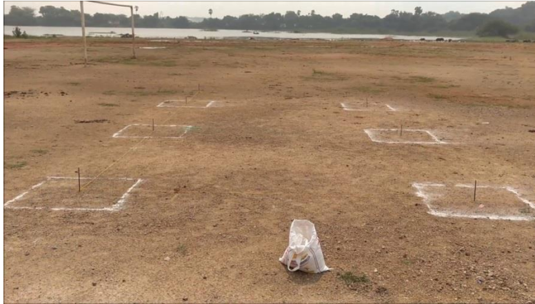
MARKING OF FOUNDATION
