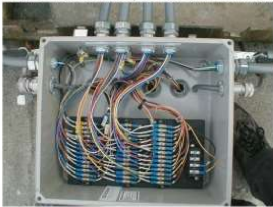
Figure 1. Traditional 4-20mA field wiring often results in a rat's nest of wires, cables and terminations.
